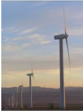
Binalood Wind Farm-Khorasan Razavi
